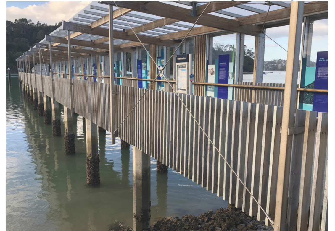
Hobsonville Point Ferry Terminal pier
