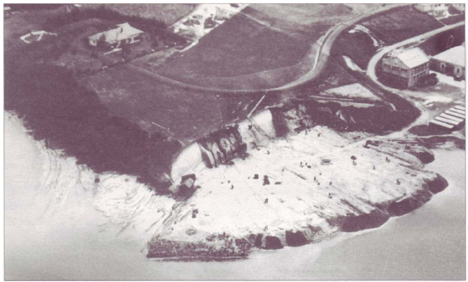
Figure 6: Cut and Fill of the Seaplane station in 1936. Note the sandstone formations in the tidal zone on the left of the photo.
