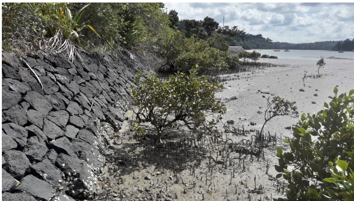
Figure 16: Retaining wall along area of proposed development.
