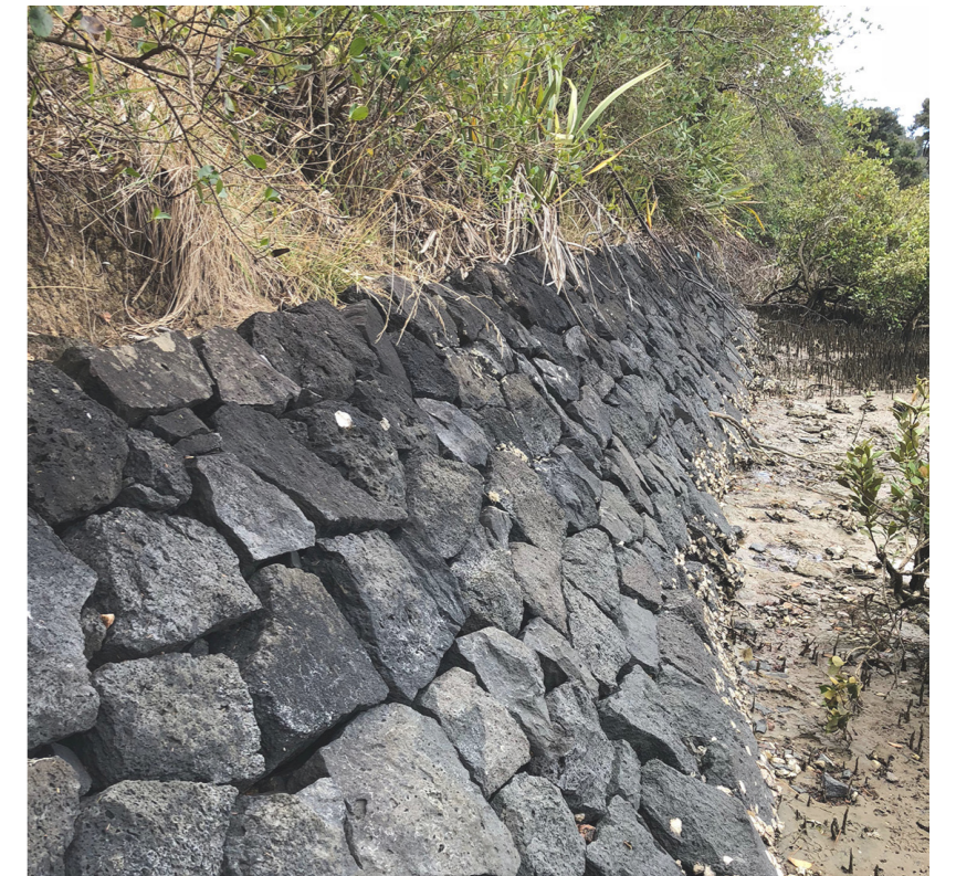
Rock sea wall at edge of site
